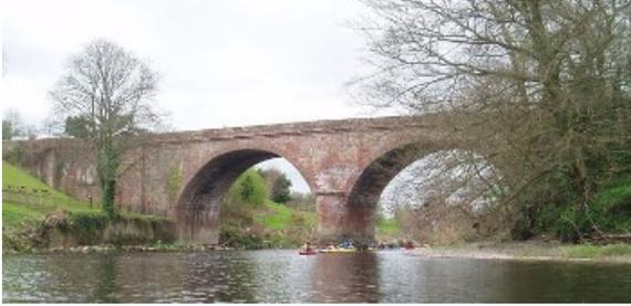
The new bridge was downstream of the previous bridge and much higher with a large embankment created on either bank to reduce the gradient of the road on each side.
