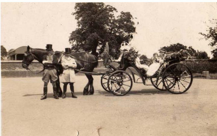
Photo taken in the School yard, looking north.
